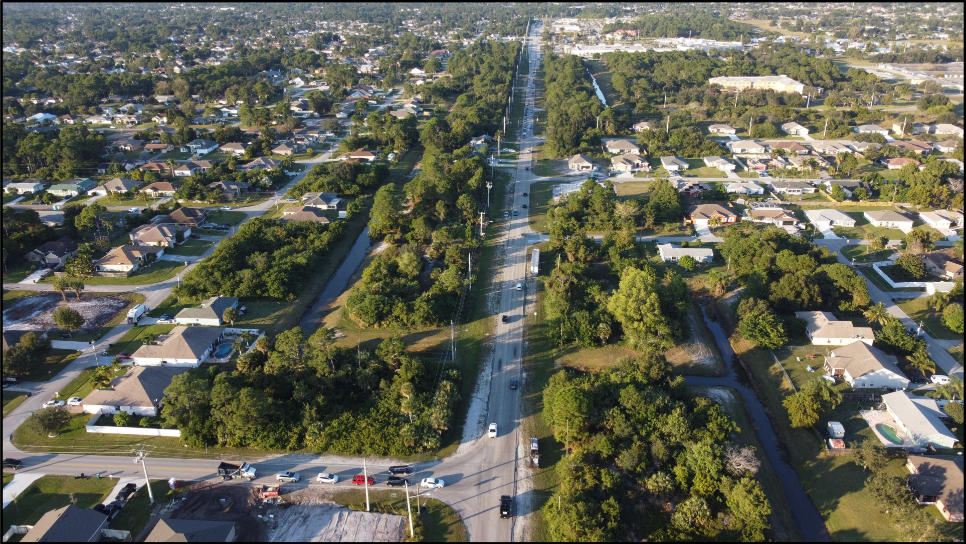
Looking north on SW Port St. Lucie Blvd. from SW Alcantarra Blvd. (pre-construction)
