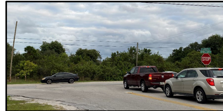
SW Alcantarra Boulevard and SW Port St. Lucie Boulevard intersection (pre-construction)
