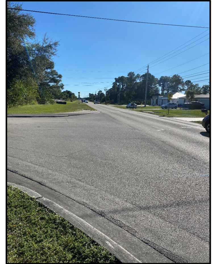
Looking south on SW Port St. Lucie Blvd. from SW Tunis Blvd. (pre-construction)
