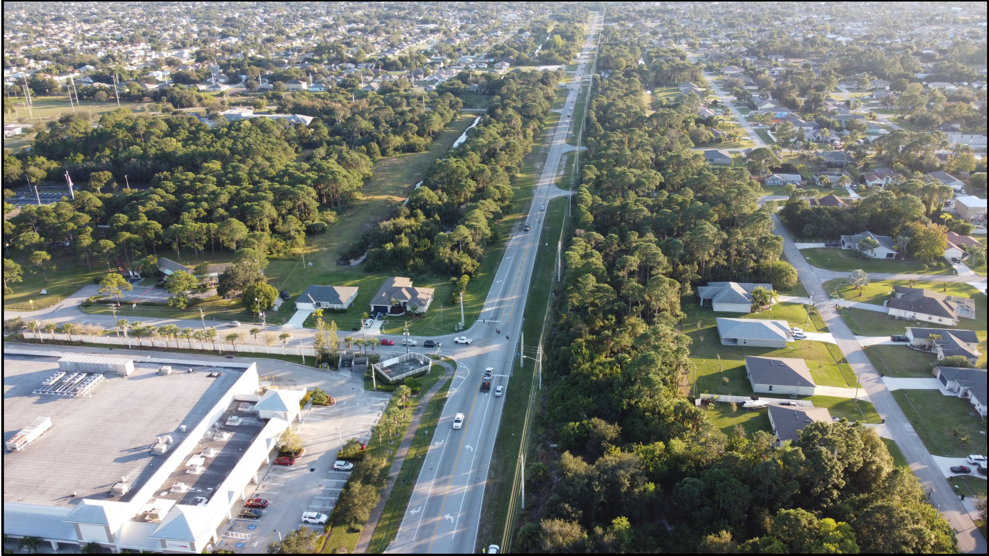
Looking south on SW Port St. Lucie Blvd. from just south of SW Darwin Blvd. (pre-construction)
