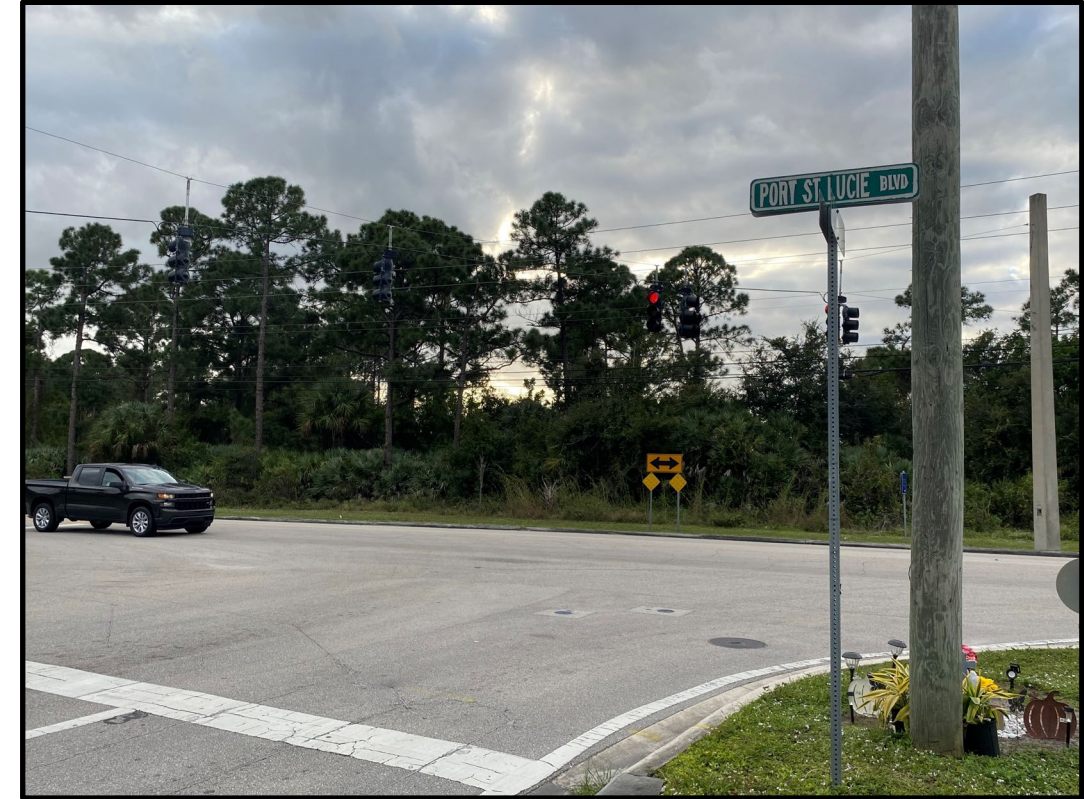
SW Port St. Lucie Boulevard and SW Tunis Boulevard intersection (pre-construction)
