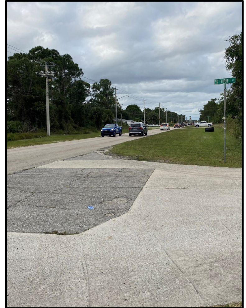
Northbound SW Port St. Lucie Boulevard (pre-construction photo)
